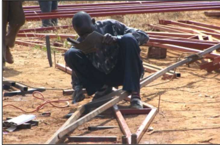
Making trussed rafters for the roofs
