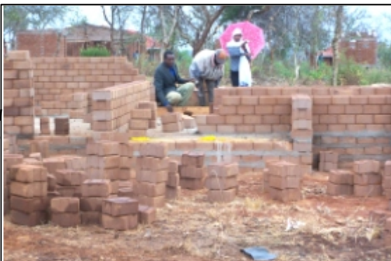
Construction of the Police Post
