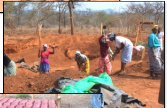
Excavation of the soil
